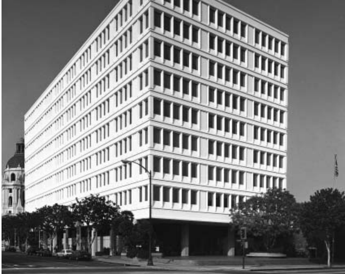
Office building owned by Wesco's property subsidiary, with Pasadena city hall in the background
